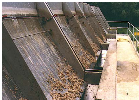
Raw municipal sewage. Stainless 554 frame - 3 x 96" and 2 x 72".
